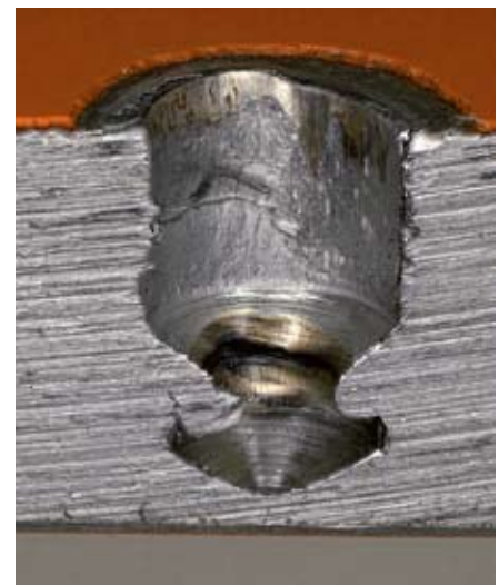
Steel base material after 7 years of exposure to sea water and pull-out of the X-BT fastener. The hole appears clean and no evidence of corrosion is visible.
