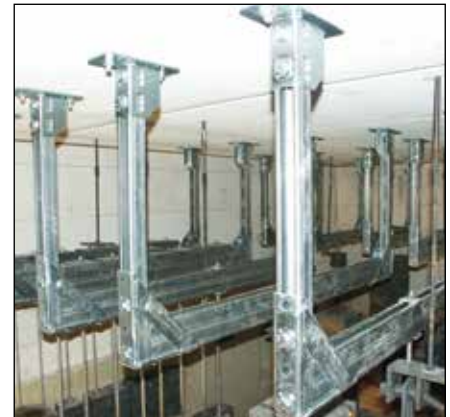
U-support with single load or multiple load before the fire test
