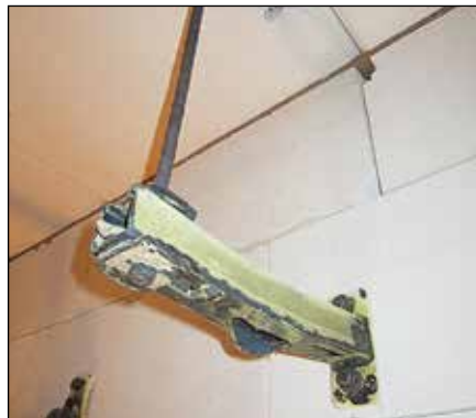
MQK bracket with central single load, after the fire test, MQA connector torn away from the channel
