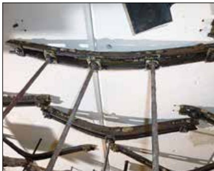
Directly-installed channel MQ-21 and MQ-41, span 700 mm
