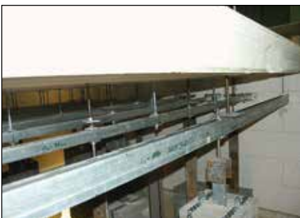
Multiple-span continuous beam with single loads, before the fire test
