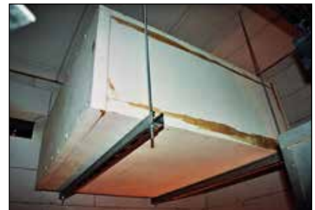
Rigid duct made from Promatect LS plates, before the fire test
