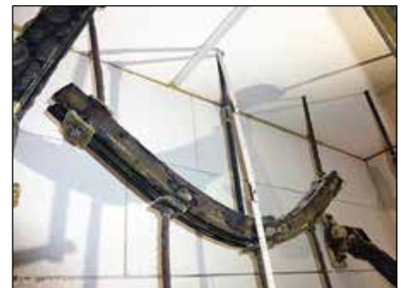
MQ-41, suspended installation, 3 single loads, MQA installed on the underside
