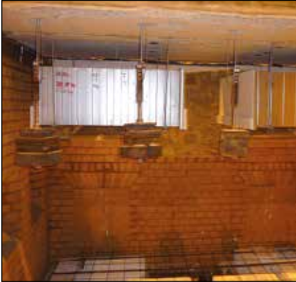
Test set-up for sheet metal ducts
